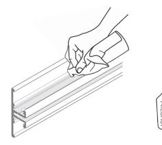
Clean the inside surfaces of the channel of dust and debris with rubbing alcohol. Dry.
